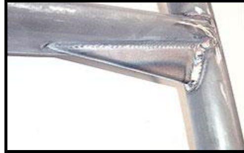
Top quality TIG welded joints
